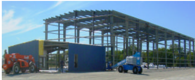
Siding at office
