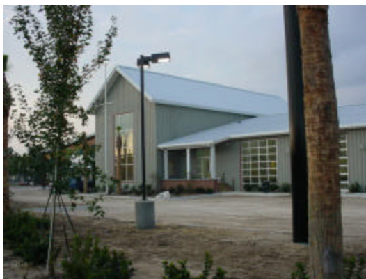
Side elevation, ready for asphalt
