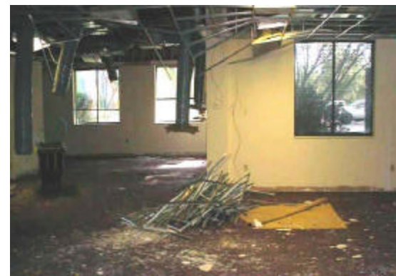
Have completed majority of the demolition on 2 nd floor
