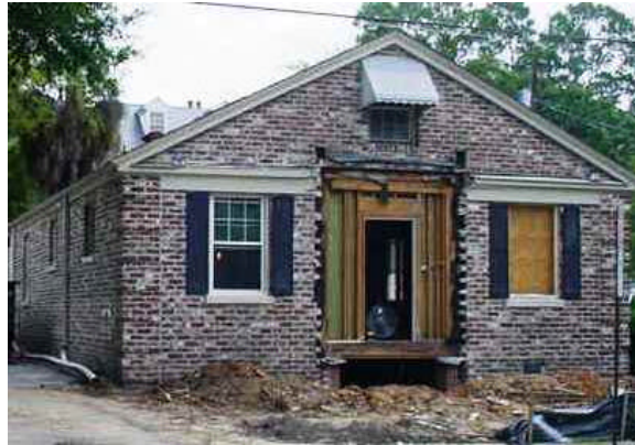
Front porch removed
