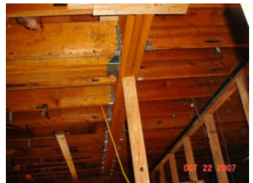
LVL in ceiling for clear span
