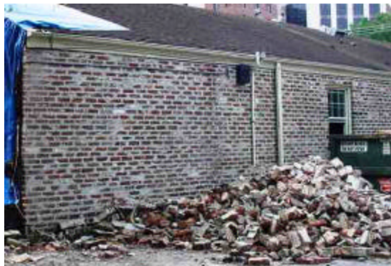
Old brick to be salvaged
