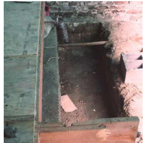
Footing for rear end wall at new drive through
